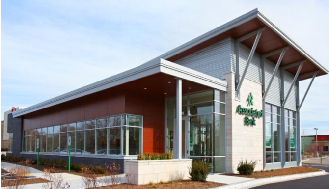
Relocated office in Waukesha, WI
