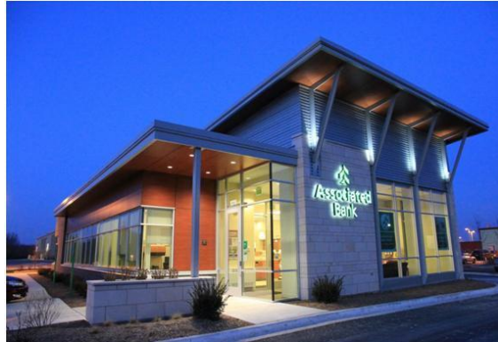
Example relocated office
