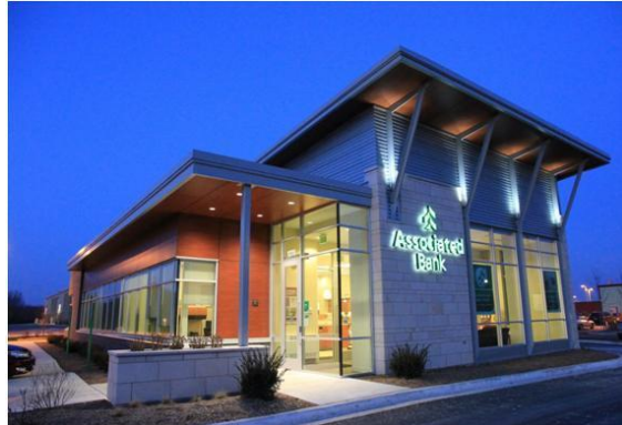
Example relocated office
